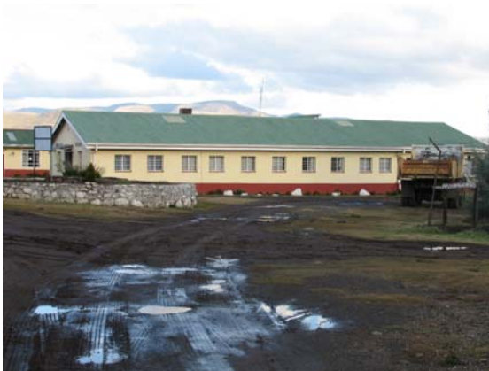
St. James Hospital in Mantsonyane, Lesotho
